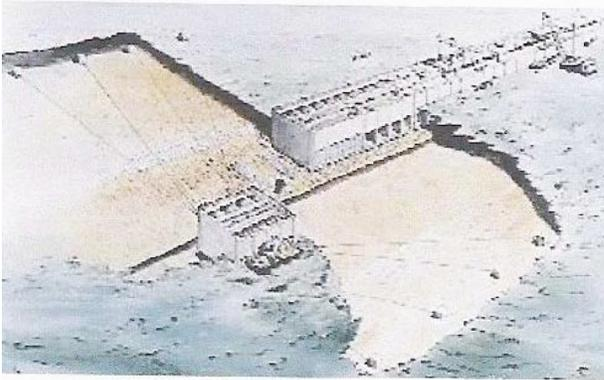
**This type of monolithic engineering structure is very inflexible in operation. Energy is also wasted by restricting the water flow through sluice gates, and the environment is damaged by the long delays imposed on the natural tidal cycle.**
