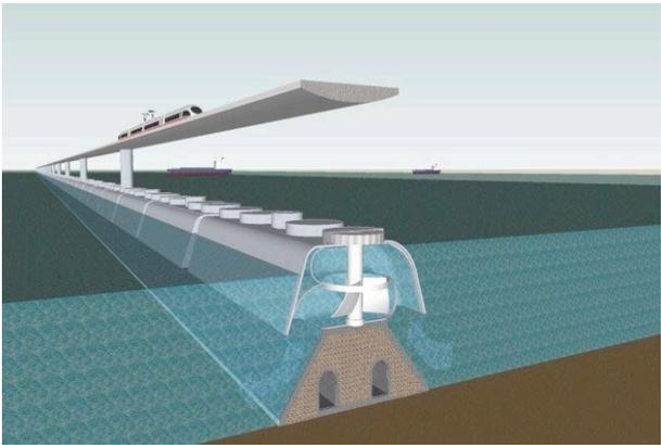
The main vertical piles of the 'Reef' structure could be extended upwards to provide support for a railway bridge, but provision would have to be made for shipping.
