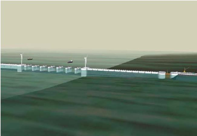
The small craft lock is shown to the right at the end of the embankment section. For illustrative purposes a section of turbine caissons is shown leading up to an island with an optional wind turbine before a section of navigation gates.
