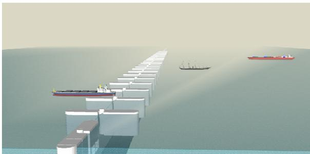
The large navigation gates that are shown in their open position, are floated into position during construction and floated to dry-dock for maintenance work.
