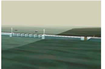
The small craft lock is shown to the right at the end of the embankment section. For illustrative purposes a section of turbine caissons is shown leading up to an island with an optional wind turbine before a section of navigation gates.
