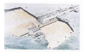
This type of monolithic engineering structure is very inflexible in operation. Energy is also wasted by restricting the water flow through sluice gates, and the environment is damaged by the long delays imposed on the natural tidal cycle.
